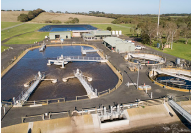
Cowes Wastewater Treatment Plant
