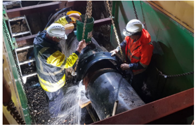
Maintenance Team doing repairs to the water main.
