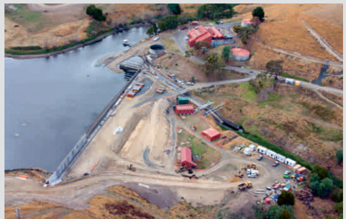
Aerial image Candowie Reservoir February 2013
