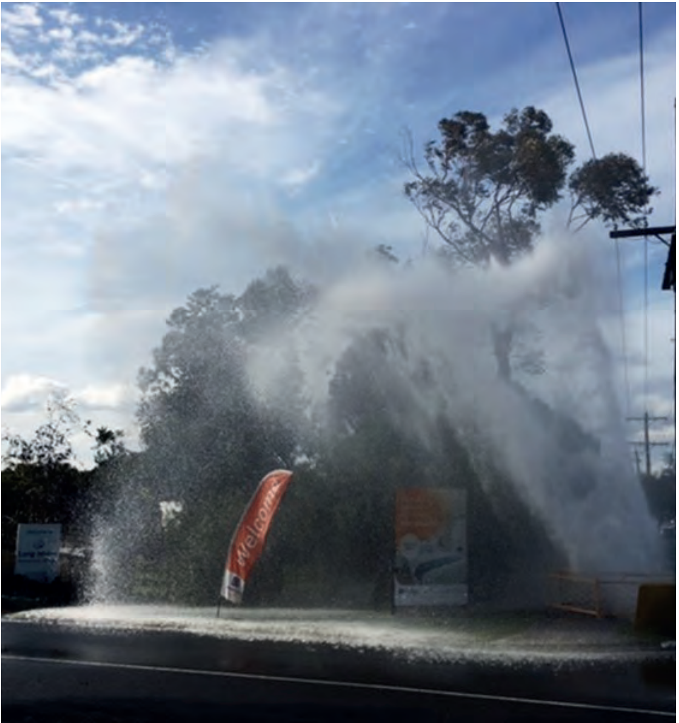
Image shows damage to a water main where the assets were not properly protected.
